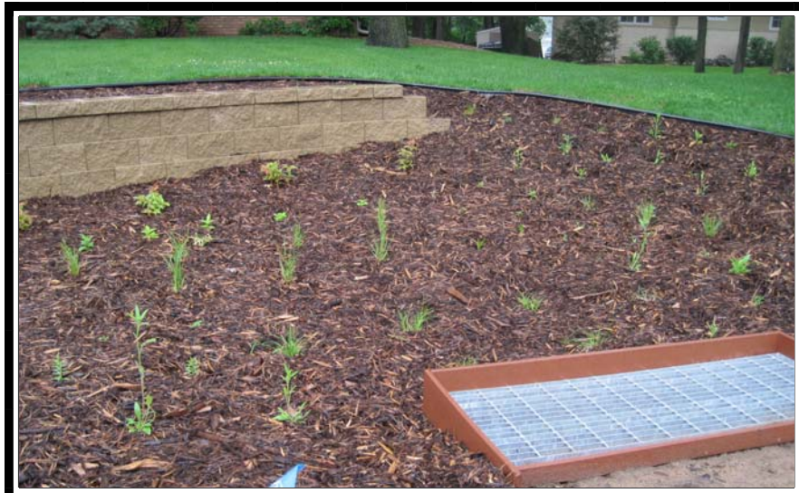
Water quality protection for the lake (in background): Rain garden (before curb cut is installed). The curb cut will be located at the inlet box which keeps soil from scouring out the area where stormwater flows in from the street).
